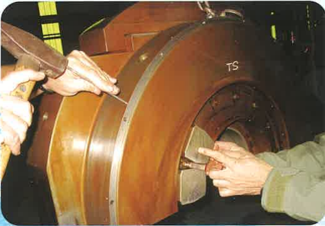
Maintenance and repairs of Pelton Turbines
