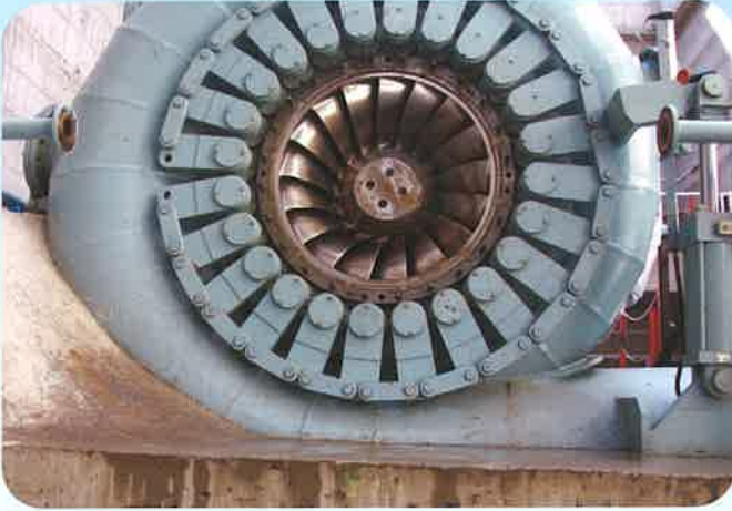
Maintenance and repairs of Francis Turbines
