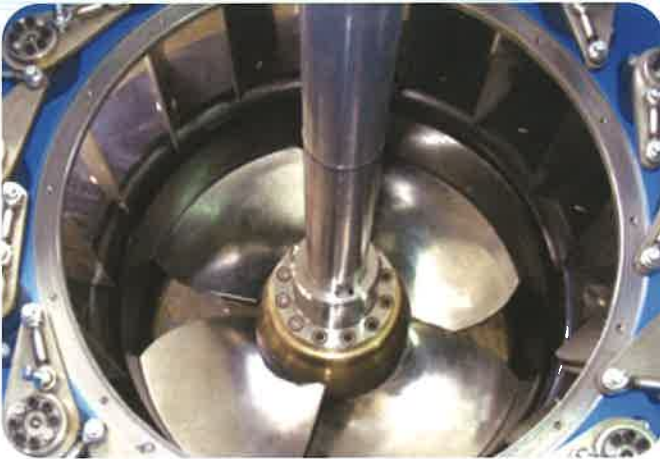
Maintenance and repairs of Kaplan Turbines
