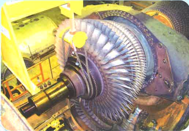
Dismantling, assmbling and commissioning
